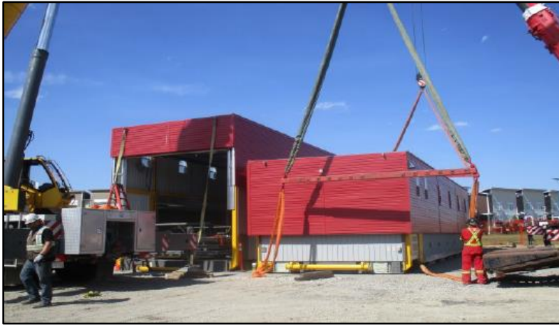
FIGURE #19: Extreme Fire Station Assembly (On-Site)
